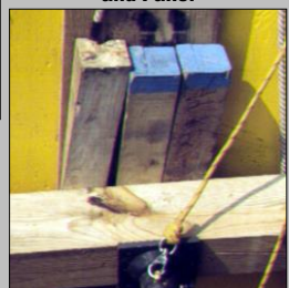
Filling Void Between Wale and Panel
