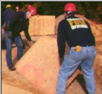
Marking Ground Pad Edges
